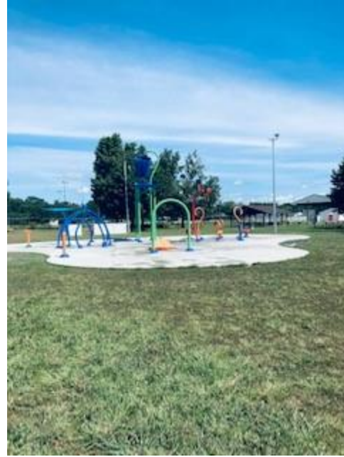
(4) Splash Pad does not have accessible pathway for use.
